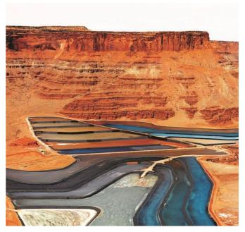
Mining tailings are often toxic, requiring treatment and remediation to ensure no harm is done to the surrounding environment. Conversion into an environmentally friendly soil is an attractive option.
