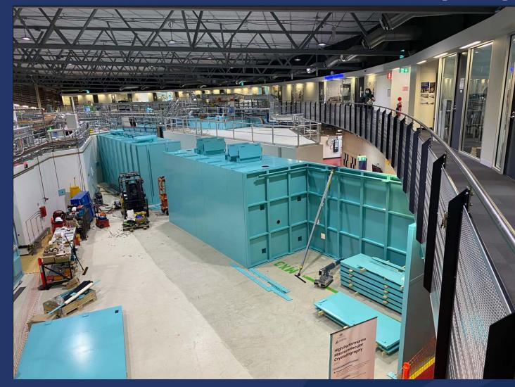
The first three shipments of the MX3 Radiation shielding hutches arrived on site from Germany late July. Hutches A and B were recently completed during the August shutdown period, well ahead of schedule. Insulation panels for hutch C are currently on-route, and completion is on track for late November.
