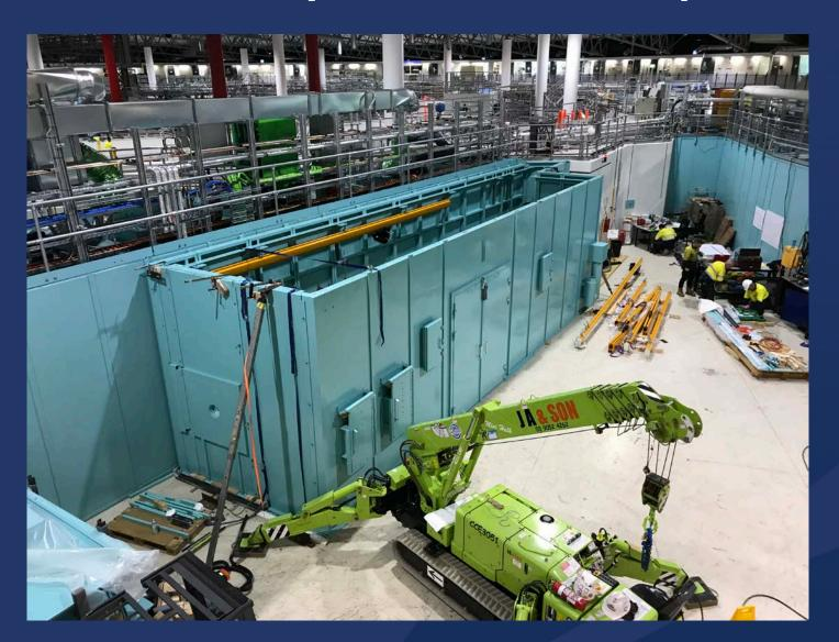
A significant milestone for the Nanoprobe Beamline with the radiation shielding for hutches A and B arriving from France in December, 2022. Hutch A is near completion, well ahead of schedule, with hutch B on track for completion by mid-March 2023.
