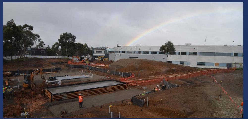
June 29<sup>th</sup> saw the pouring of the 900-mm thick endstation slab, designed to resist environmental vibrations and enable NANO to reach a 60 nm resolution.
