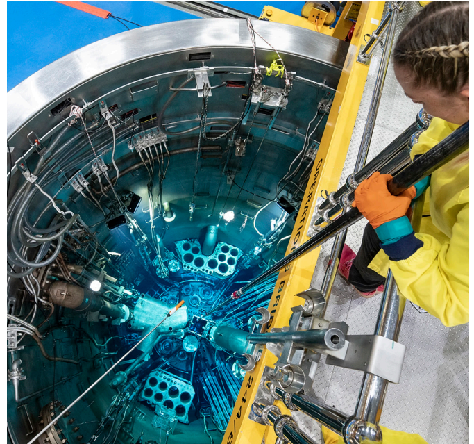
The OPAL research reactor at ANSTO.
