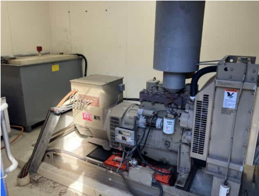
Photograph 19: Standby generator on first floor with above ground storage tank in background (photo supplied by ANSTO) Photo direction: Not applicable
