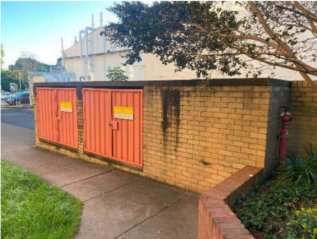
Photograph 3: Enclosure for the gas meter (left) and water meter (right) station at the east side of the building. Both doors are secured with padlock and signages posted.
