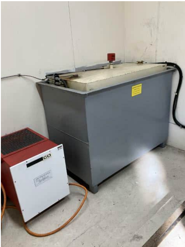
Photograph 20: Diesel above ground storage tank for standby generator (photo supplied by ANSTO) Photo direction: Not applicable
