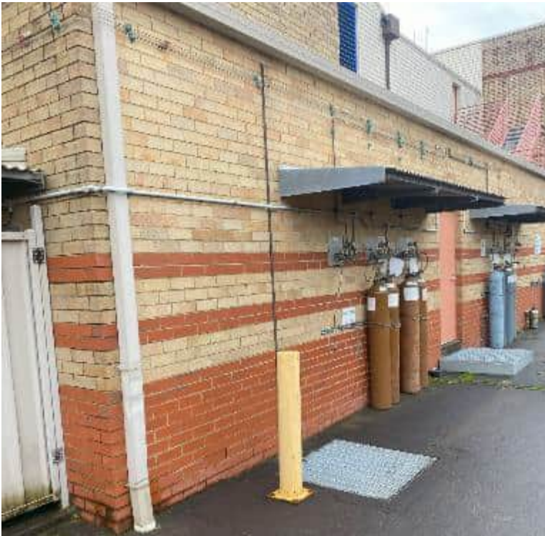
Photograph 9: Flammable and non-flammable gas cylinders secured in chains inside the fenced area at the south side of the building.
