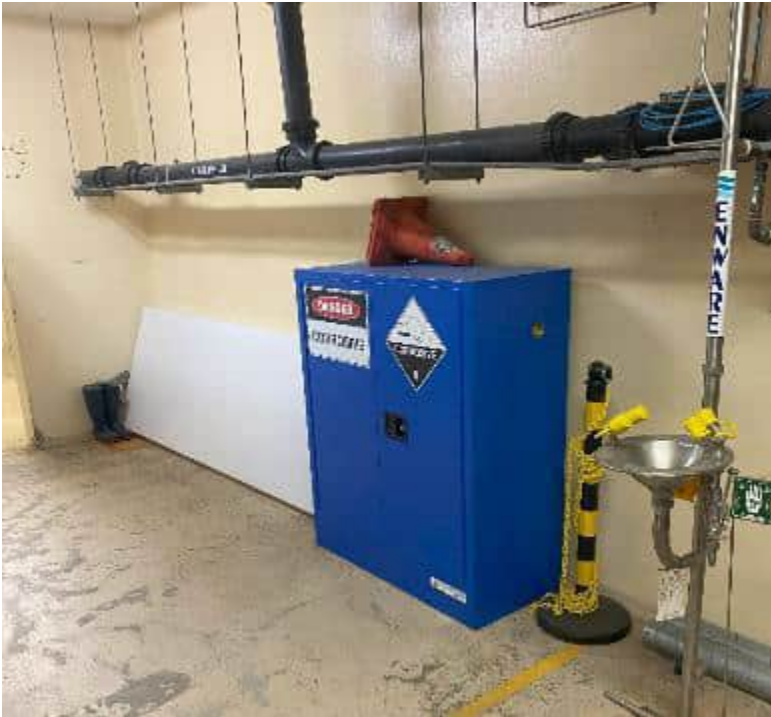
Photograph 13: A chemicals cabinet for corrosive chemicals at the basement of the building. An eye washing station is adjacent to the cabinet in case of emergency.
