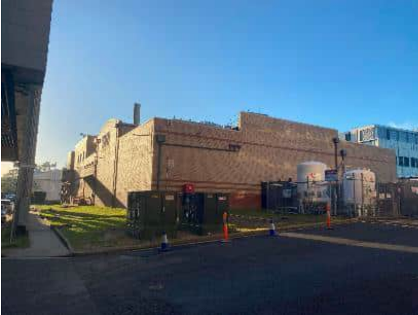
Photograph 1: A view of the western and northern side Building 81, NRCF (the Site) across Hospital Road. The Site features two pressurised aboveground storage tanks (ASTs) containing liquid nitrogen and two electrical utility enclosures at the southwestern corner of the building. The ASTs are for an adjacent property and not used by ANSTO.
