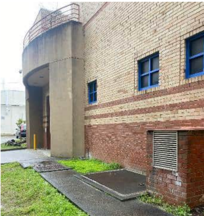
Photograph 14: Drainage steel cover and steel grates at the northern side of the building. The cover close to the façade is to enable access to the basement for bulky items.
