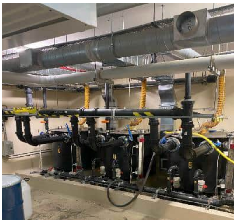
Photograph 11: Bunded trade waste collection system located at the basement.
