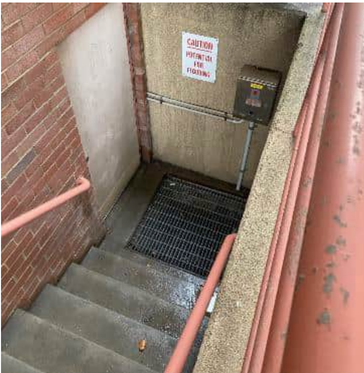
Photograph 10: Stairs leading to the basement of Building 81. A large steel grate is located at the landing area and a signage that cautions about the potential for flooding. The steel grate is for a sump to pump out stormwater.
