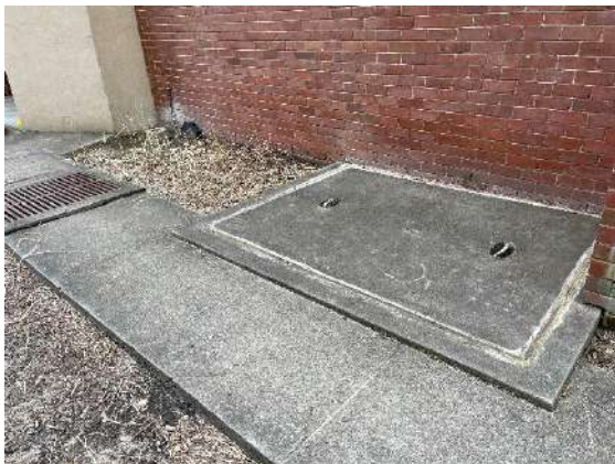
Photograph 02 View of eastern stormwater drain and manhole in northern nature strip as viewed from the north.
