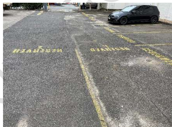
Photograph 05 View of eastern carpark as viewed from the south
