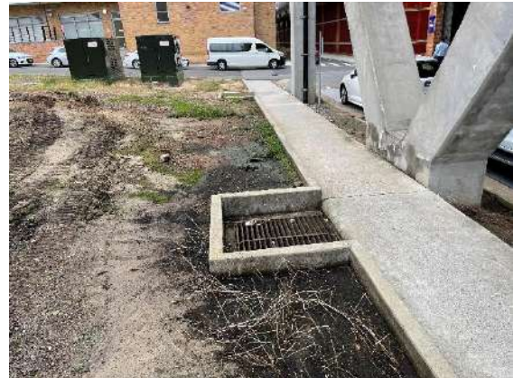
Photograph 04 View of western stormwater drains in northern nature strip as viewed from the east.
