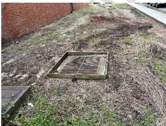
Photograph 03 View of central stormwater drain in northern nature strip as viewed from the east.
