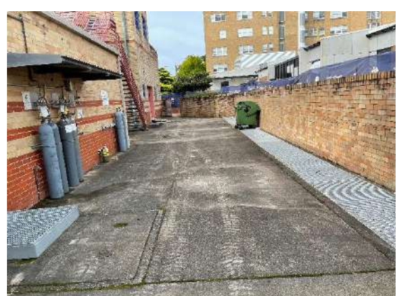
Photograph 06 View of southern exterior hardstand area as view from the west.
