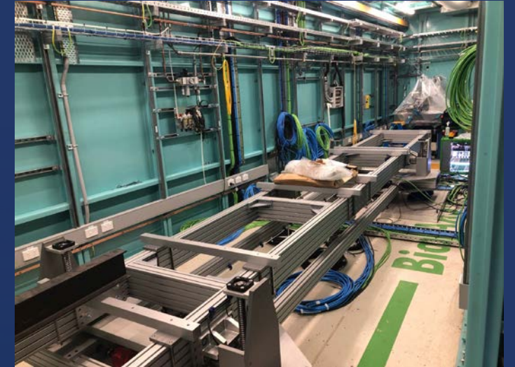
BioSAXS - Utilities installation & Endstation construction
