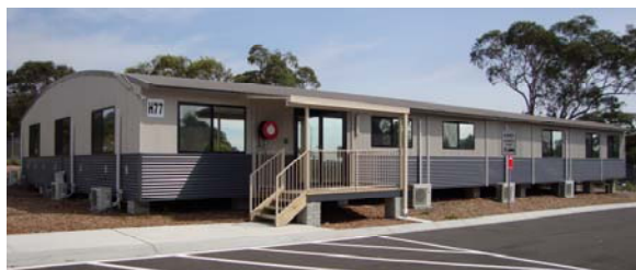
NBI-2 Project Home – Building Hut 77
