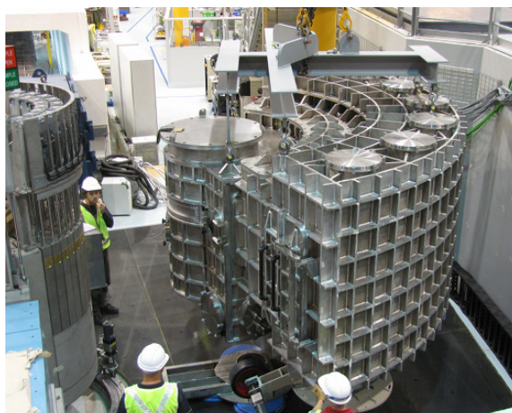
The Pelican vacuum tank being manually guided into position on its dancefloor.
