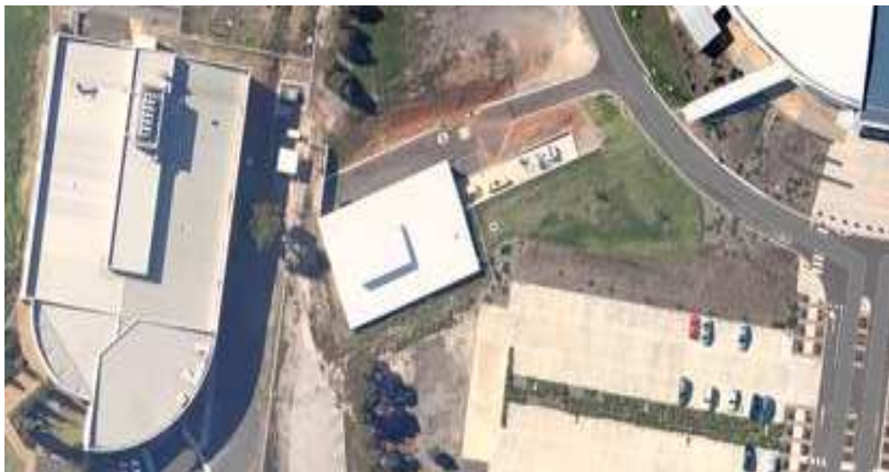
The IMBL and SAT building with the Biomedical Imaging Consortium building (left)
